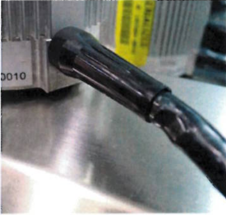
Figure 5: Cable Damage at the Motor Bend Relief
